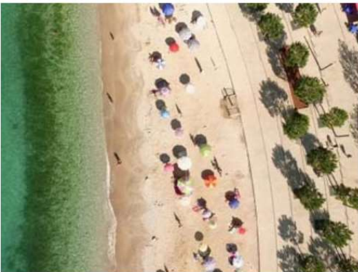
Renovation of the Himarë Waterfront
