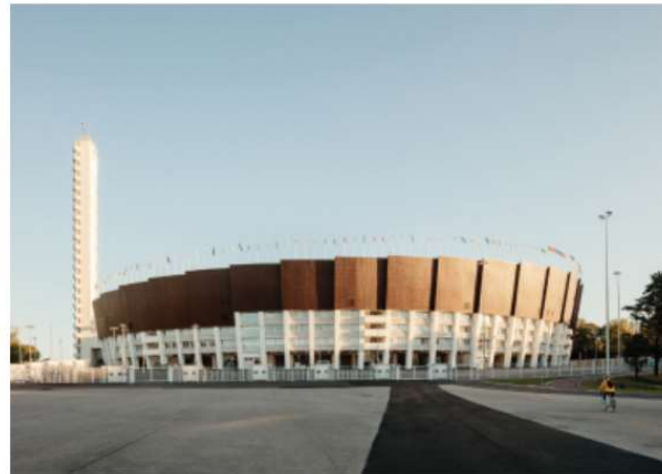
Helsinki Olympic Stadium Refurbishment ... K2S Architects Ltd, Arkkitechdit NRT Helsinki, Finland
